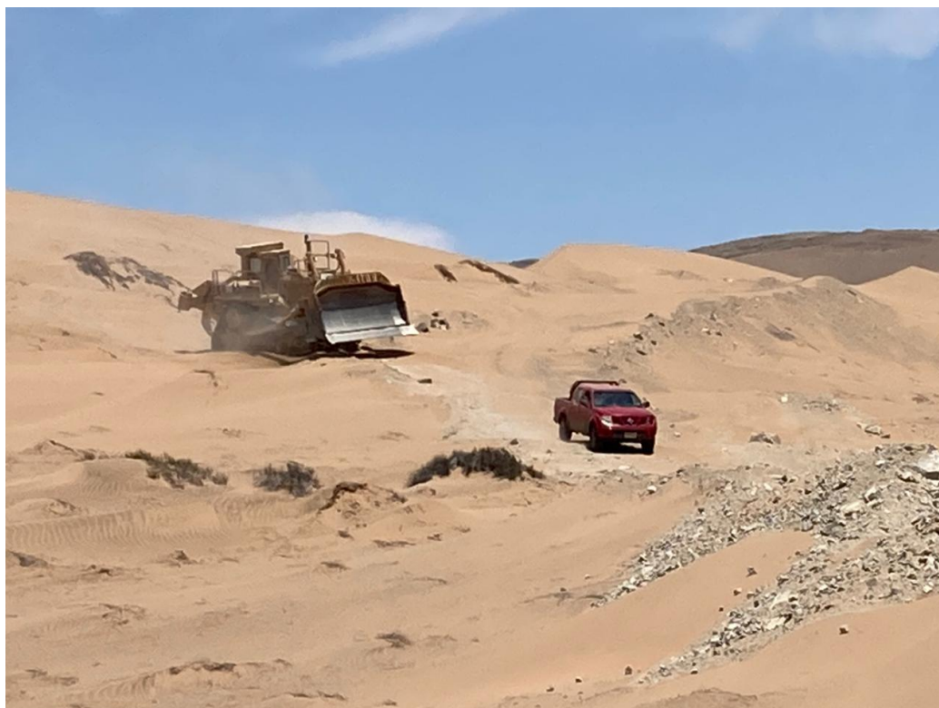
Figure 2: Commencement of drill road and diamond drill pad construction Algarrobo Project.
