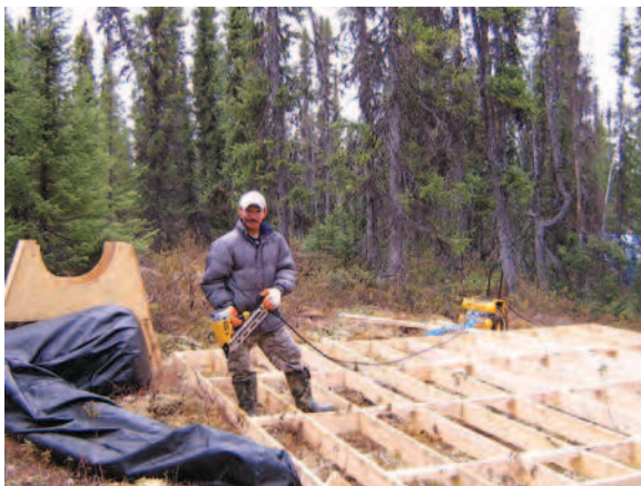
Carpenter Saunders, of Kuujjuaq, erecting the field infrastructure.
